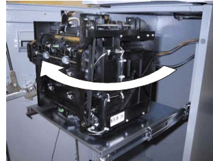
Rotate mechanism to service position.
